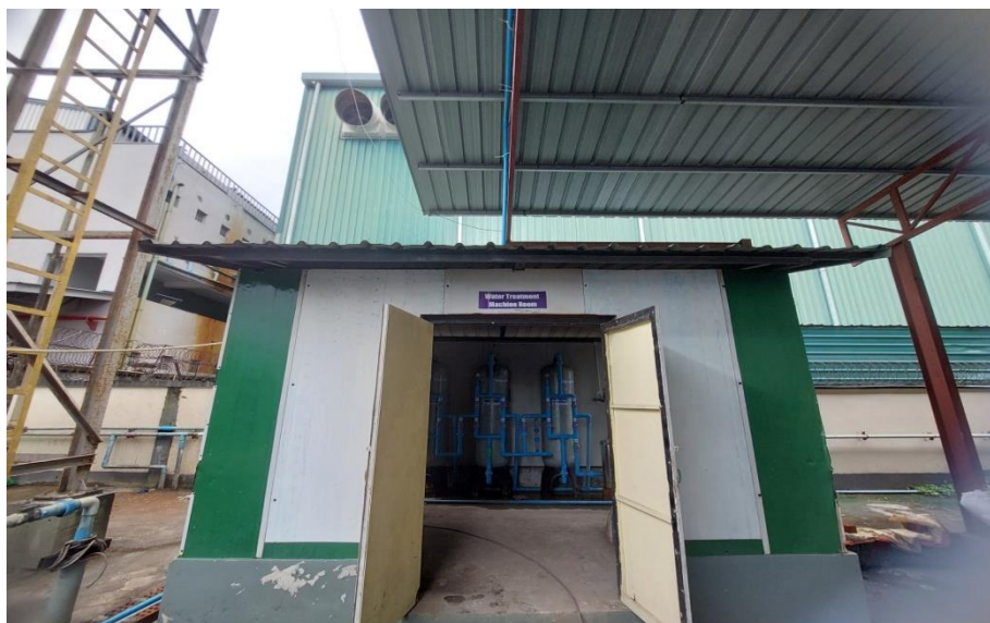
Figure 3-9 photographs of water treatment plant
