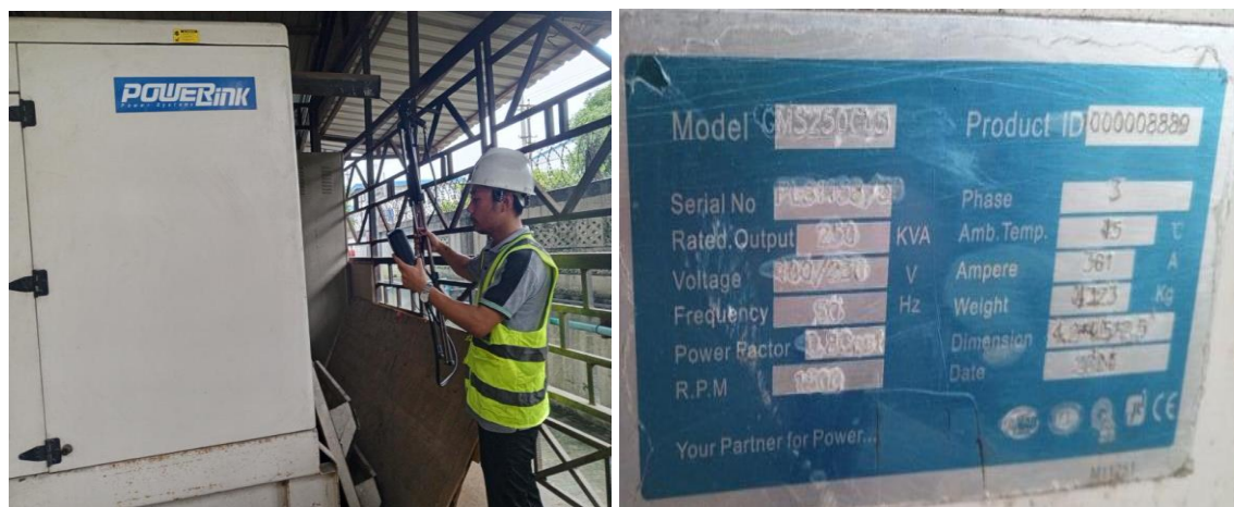
Figure 4-31 Photograph of electric generator stack emission
