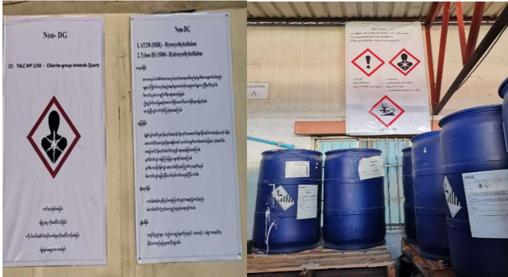
Figure 3-5 Chemical storage condition, attached SDS
