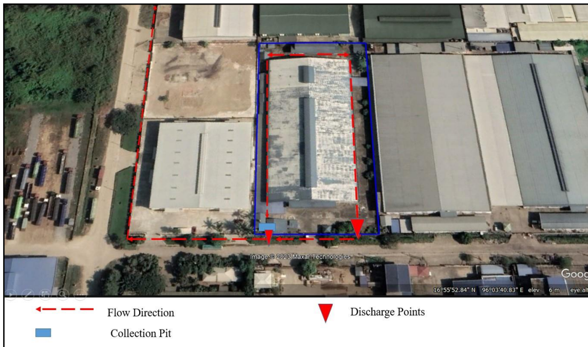
Figure 3-16 Drainage Channel Photo
