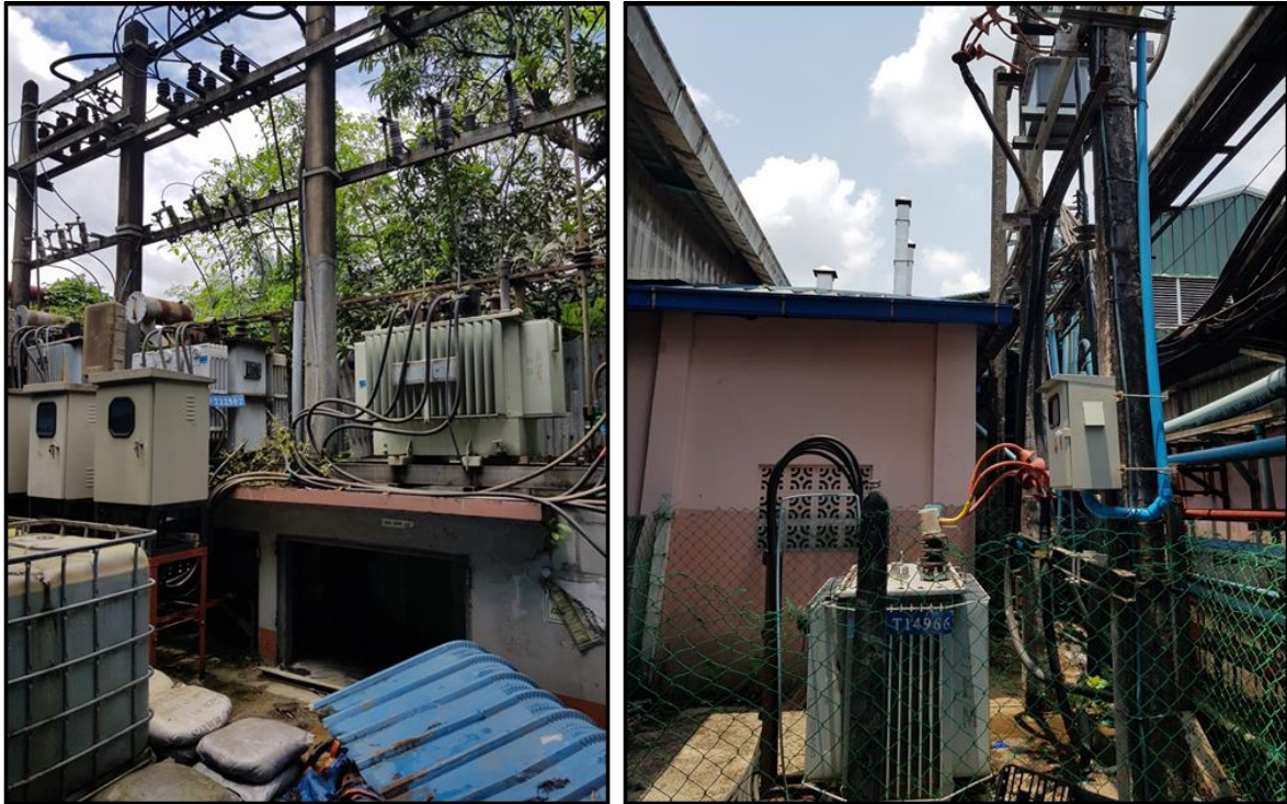
Figure 3.15: Transformer
