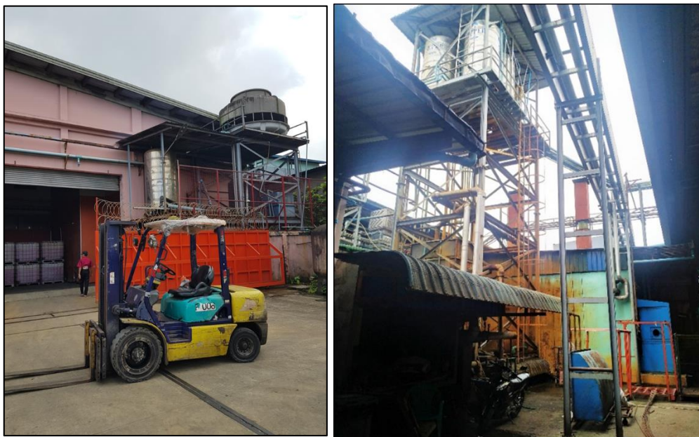
Figure 3.14: Water Storage Tank
