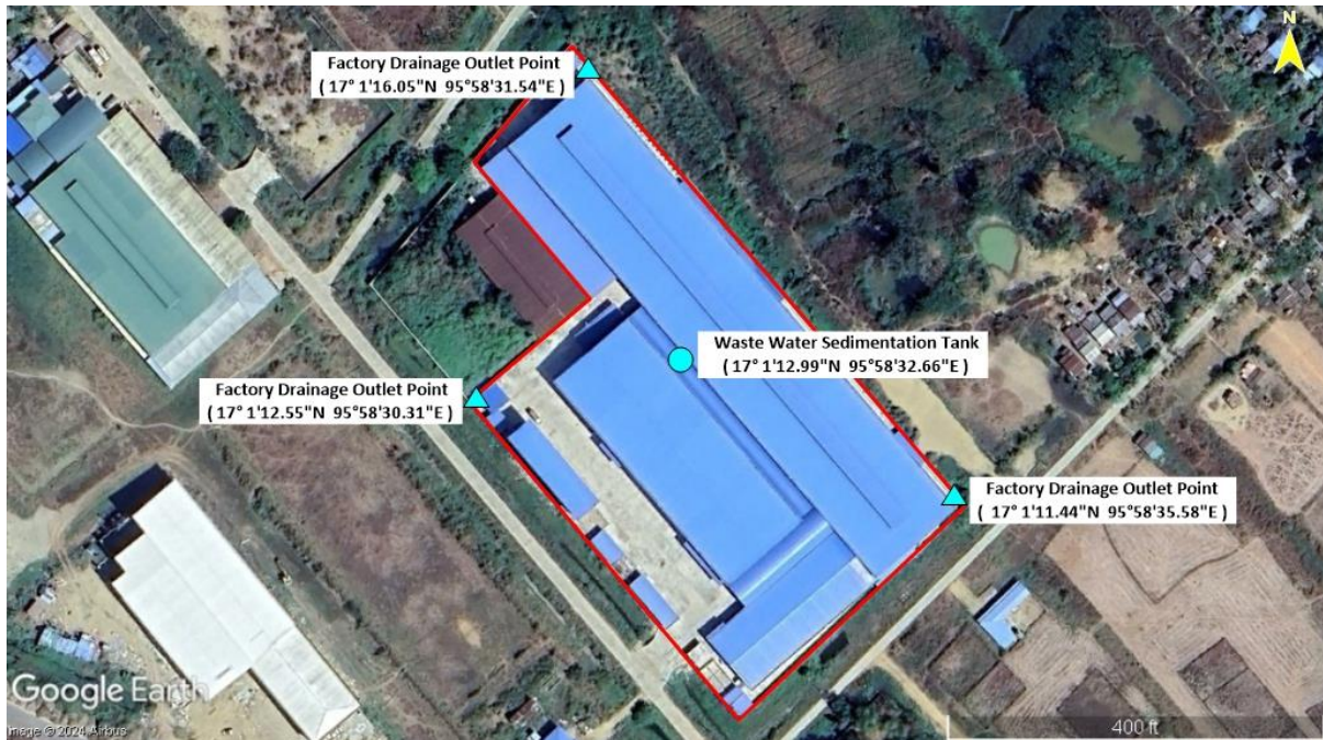
Figure 6.7 Factory Drainage and Outlet Point of the Factory Drainage
