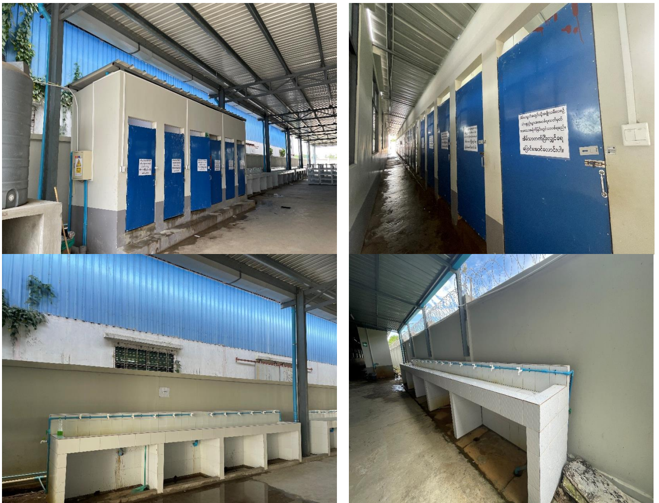
Figure 3.22 Toilet Facility Photo
