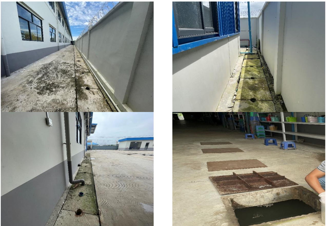
Figure 5.3 Drainage System and Sedimentation Tank in the project area
