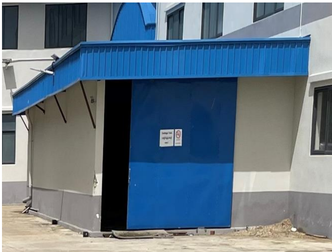
Waste Storage Area
