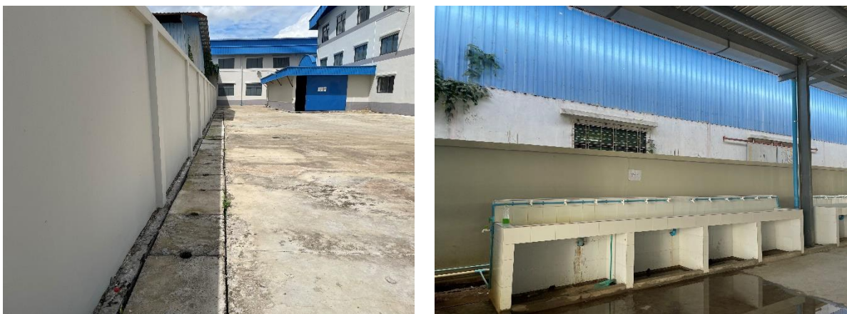
Figure 3.20 Drainage System and Hand Washing Basin
