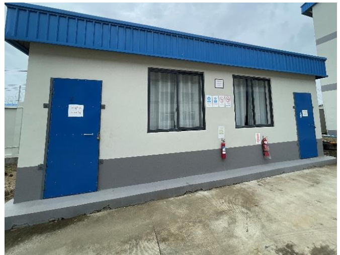
Hazardous Waste Storage Area
