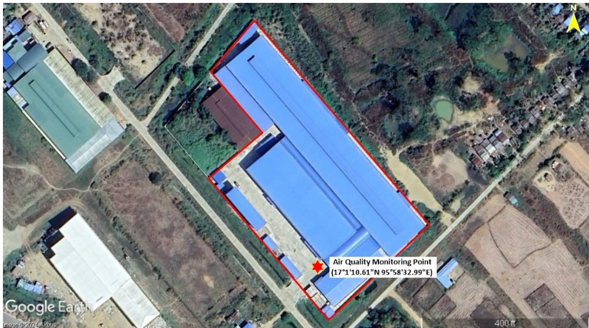
Figure 6.3 Air Quality Monitoring Point
