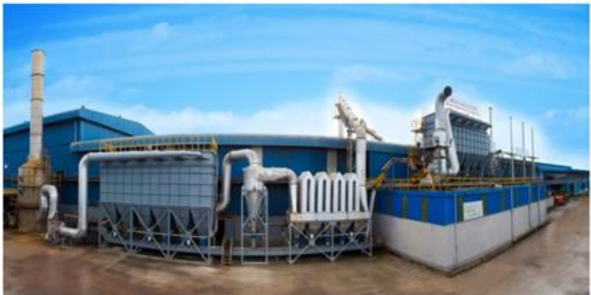
Figure 3-23 Air Pollution Preventing System
