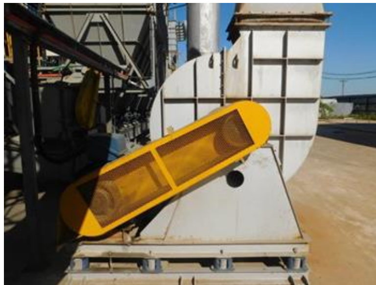
Figure 3-27 Dust Line, Blowing Fan and Motor
