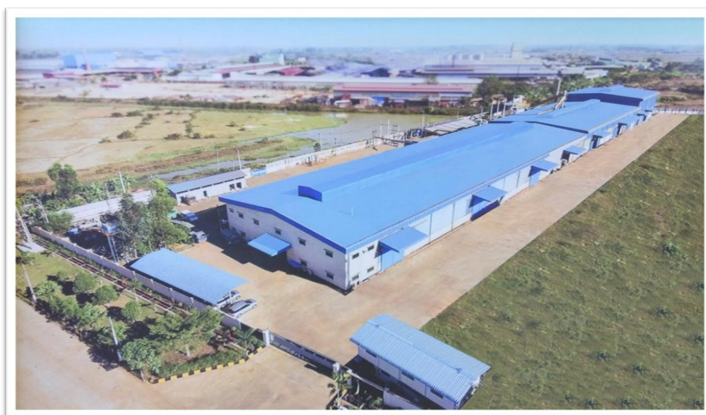
Figure 3-1 Lead Smelting and Refinery Factory, Yangon Metal Industry Co., Ltd
