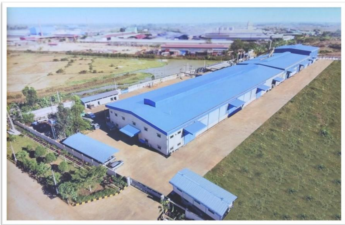
Figure 3-2 Lead Smelting and Refinery Factory, Yangon Metal Industry Co., Ltd.
