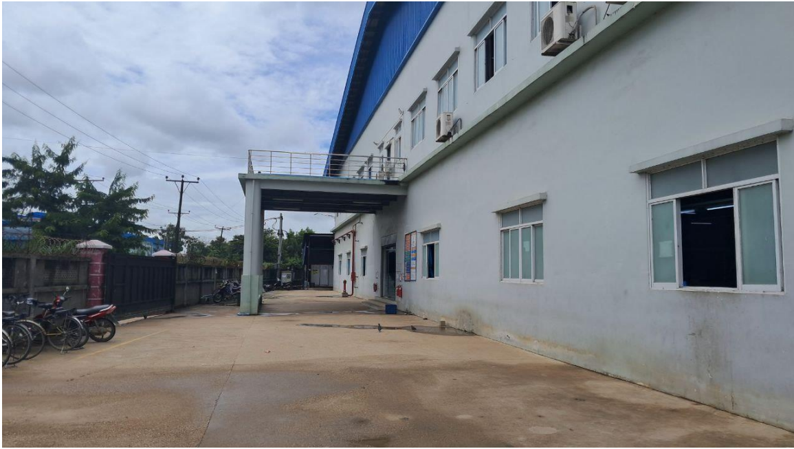
Air Conditioners and Exhaust Fan
