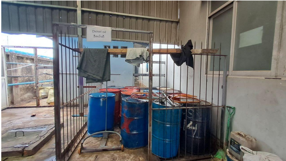
Figure 4-12 Fuel Storage Room
