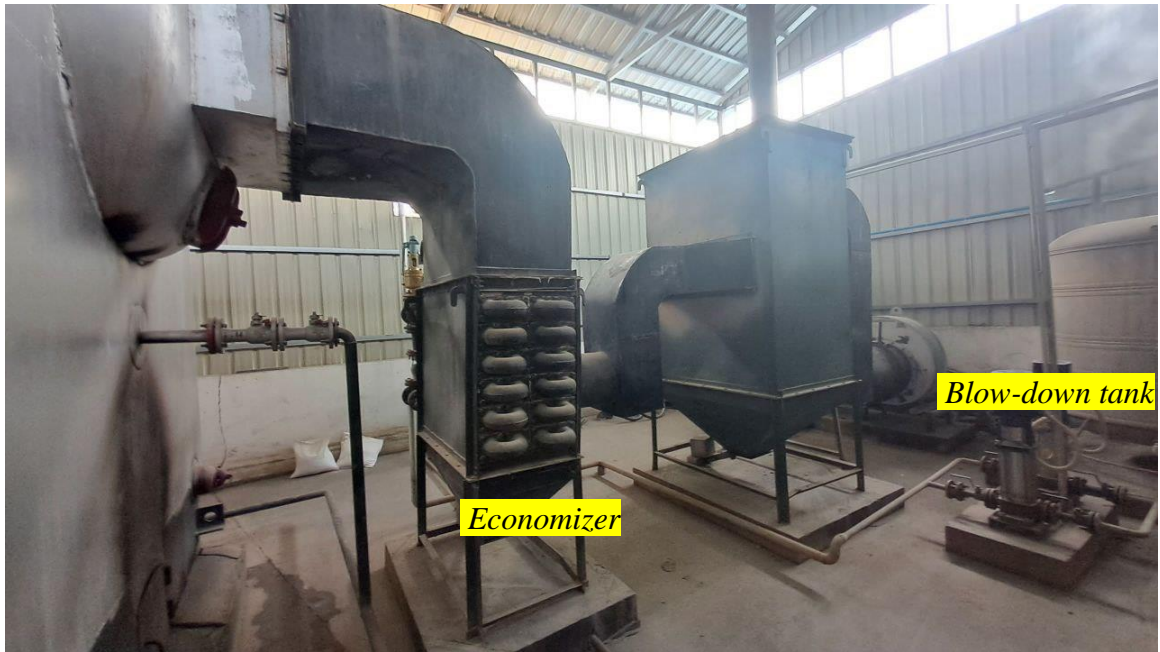
Figure 4-14 Boiler Dust (Fly Ash) Control System
