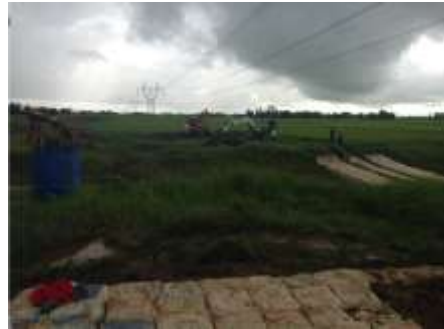
Excavation work at the site in the morning
