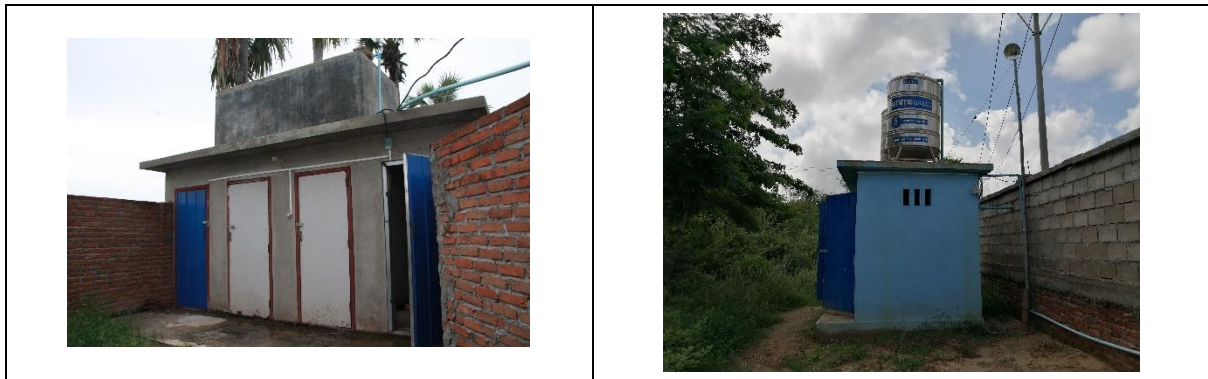
Figure 3-33 Photos of Sanitary Facilities
