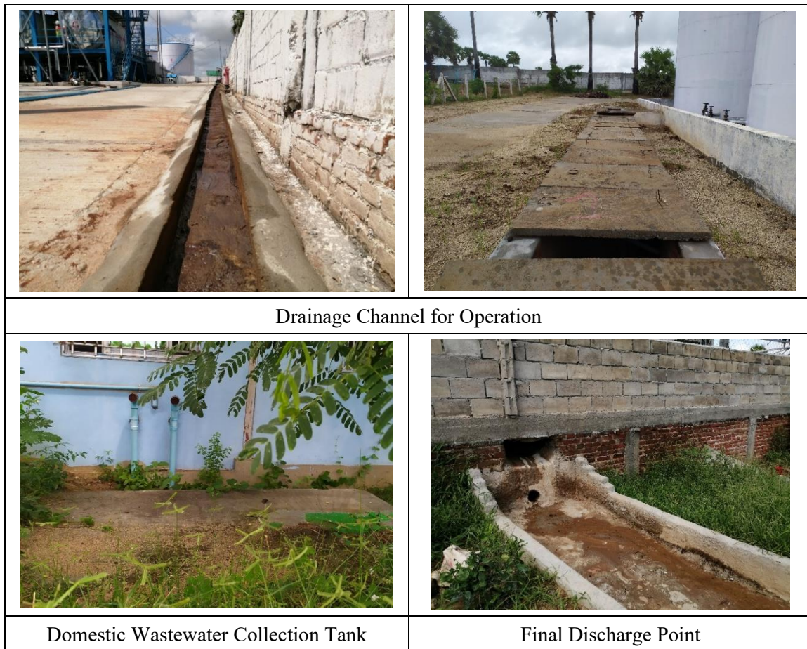
Figure 3-26 Drainage System for Domestic and Operation Wastewater
