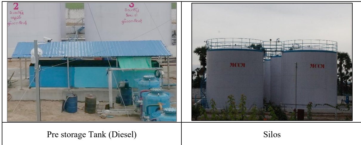
Figure 3-13 Final Product Storage
