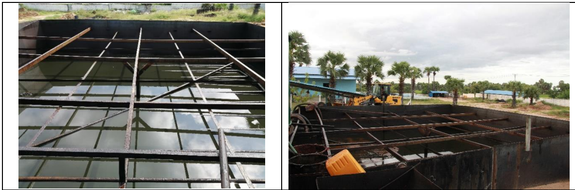
Figure 3-5 Heating Crude Oil in Preliminary Tank
