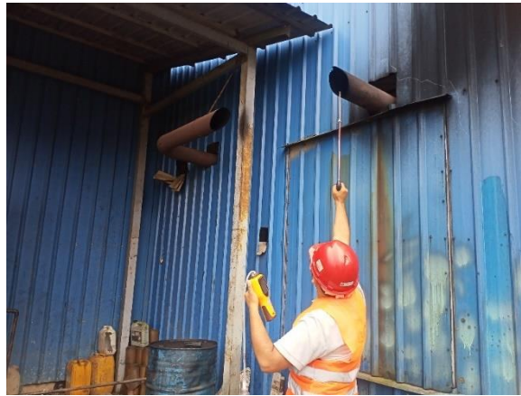
Figure 6-9 Generator Stack Emission Measurement Activity
