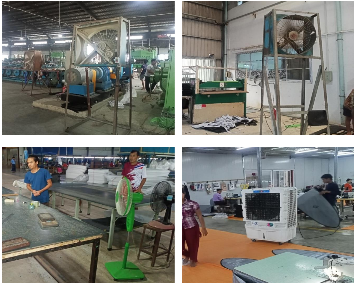
Figure 2-19 Ventilation Supply Photo
