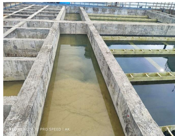
Photo 3-8: Clearing water layer by layer
