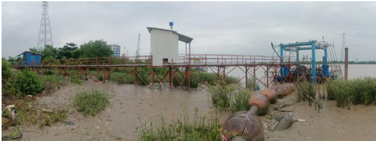
Photo 3-6: Place of Intake structure
