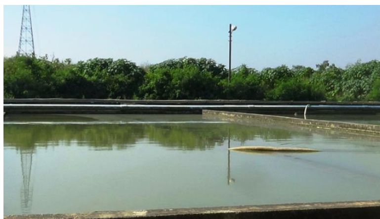
Photo 4-24: Showing the vegetation of the back View of Power Plant
