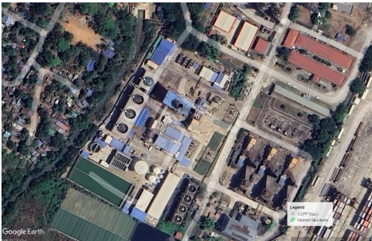
Photo 3-32: Ahlone Power Plant and nearest infrastructure in vicinity
