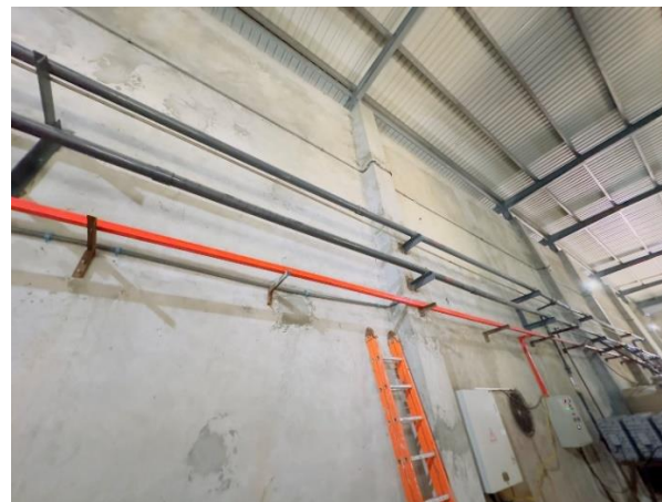
Photo 3-25: Exit pipelines from mix-ion column
