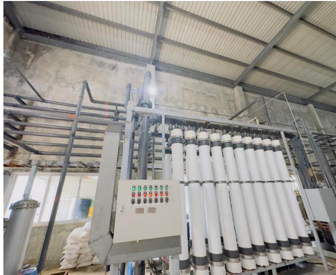
Photo 3-19: Ultrafiltration system
