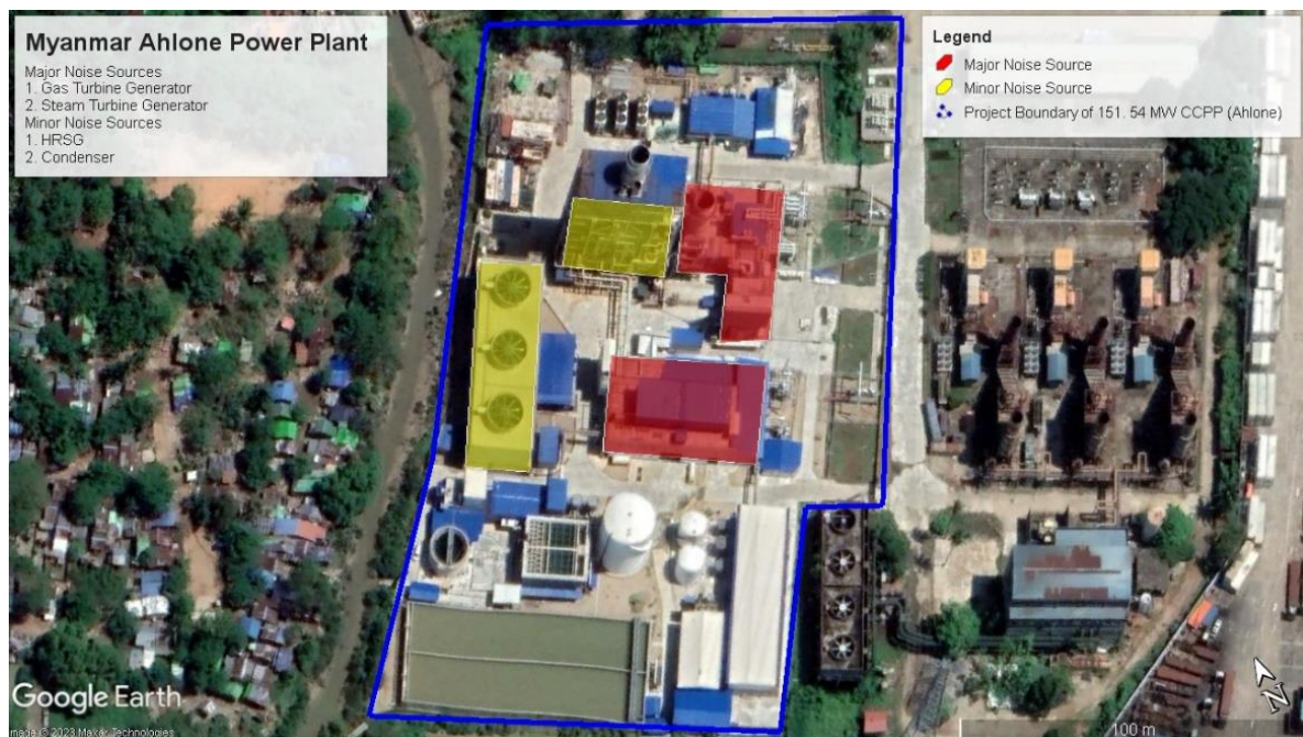
Figure 5-2: Noise Sources within 151.54 MW CCPP Project Boundary
