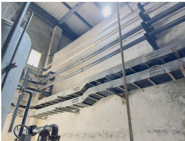
Photo 3-25: Exit pipelines from mix-ion column
